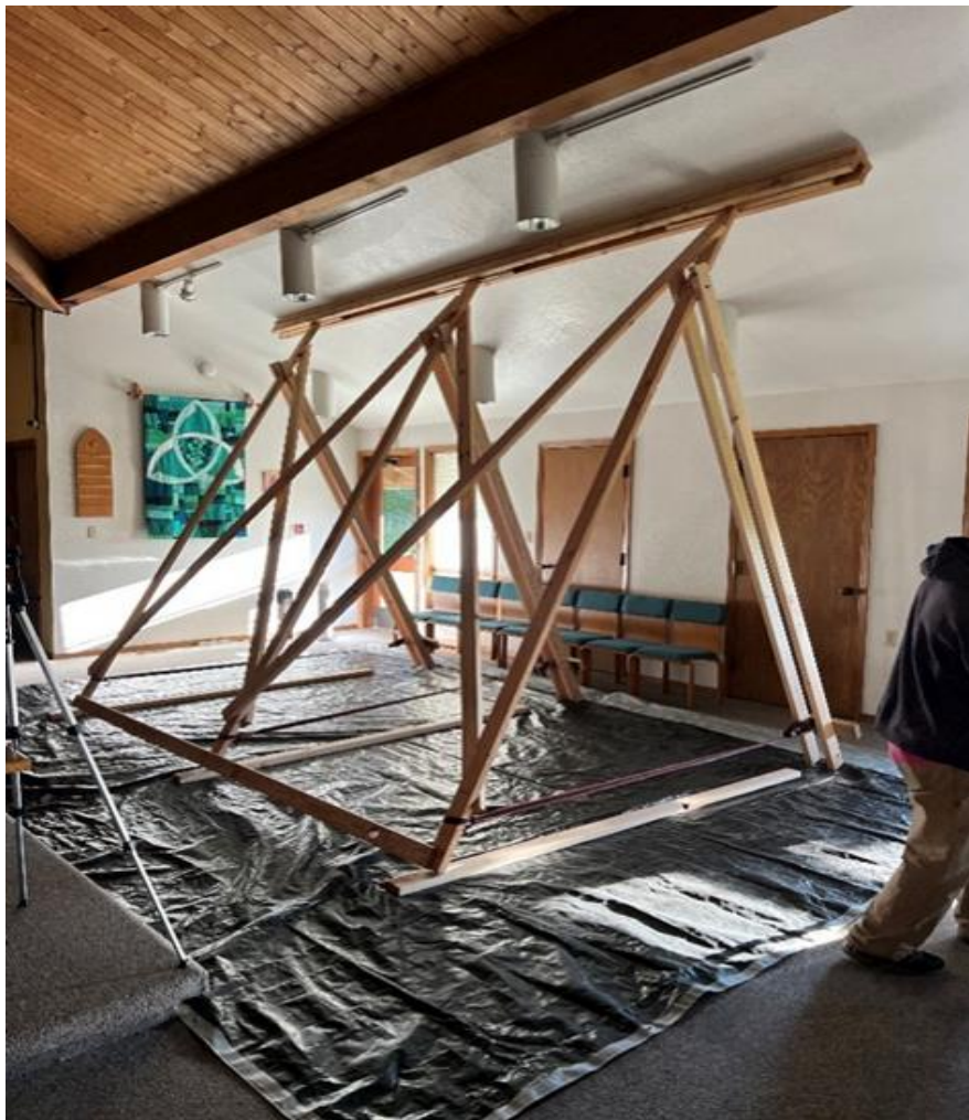
Figure 3 Rafter support frame supporting the rafters during temporary repairs
